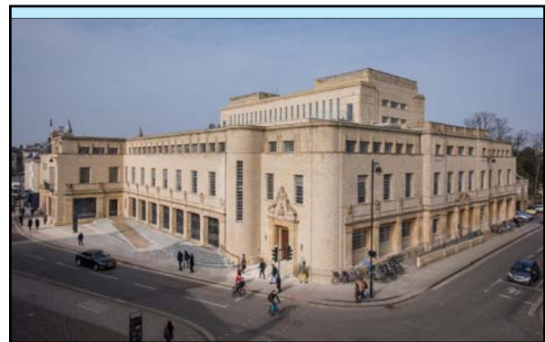
The Weston Library (opened 2014): across Broad Street from the Old Bodleian Library
